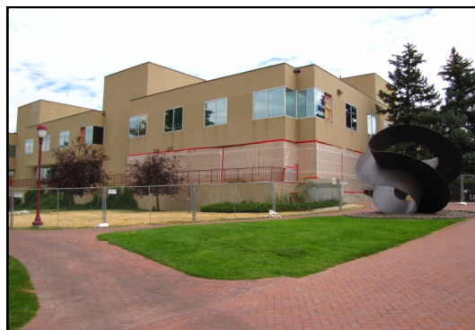
Construction continues on Penrose Library.
