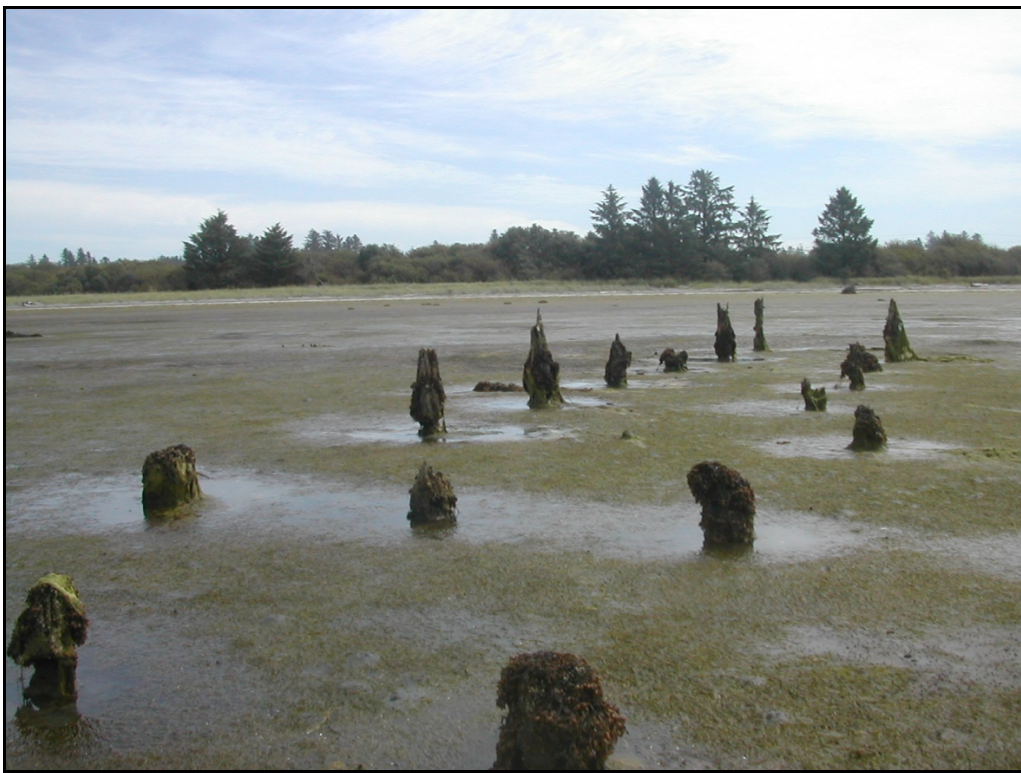
Figure 45: Ocosta Docks, August 2008.
