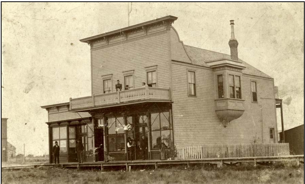
Figure 29: High false front parapet disguises the simpler structure behind this Ocosta Store, 1890-1920, Polson Museum Collection.
