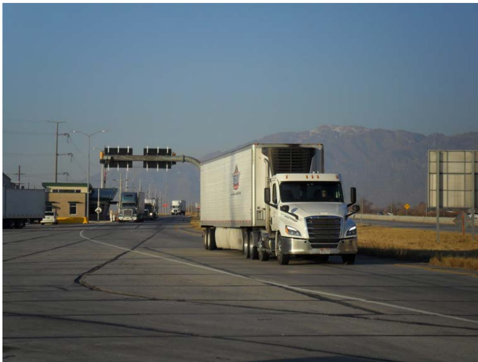
Figure S3. View looking north toward the scales showing the Port of Entries lane arrangement. Speed limits through the port were 3mph on the west lane (left) and 20 mph on the east lane (right).
