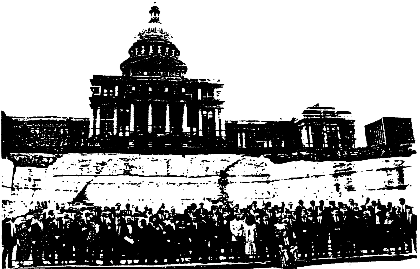
Making sure that they all fit, the Texas Legislature posed in the giant hole that has become offices for 99 House members and 10 senators, as well as committee rooms, an auditorium, a cafeteria and parking for 650 vehicles. Tunnels connect the underground complex to the historic Capitol.
