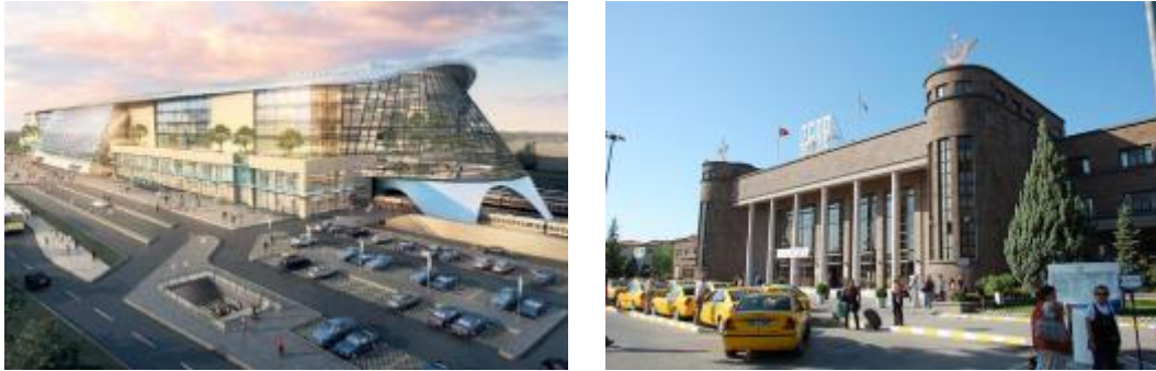
Figure 2. The older Ankara Railway Station versus the new Ankara Train Station (Hsu, 2008; RailTurkey, 2016).
