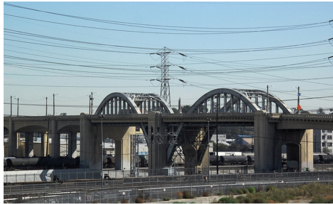
Figure 1.1. A picture of the old Sixth-Street Bridge. Photo taken from Caltrans' 6 th Street Viaduct seismic improvement project.
