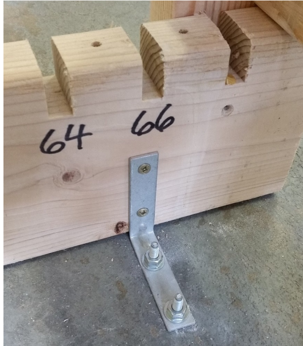
Figure 5.3: Anchor bolts and steel bracket securing each corner of the experimental apparatus to the concrete floor.
