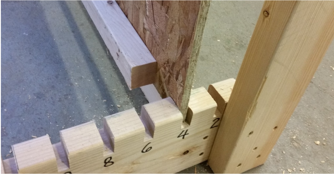
(a) Wall rests in routed slots in the base cross beams
