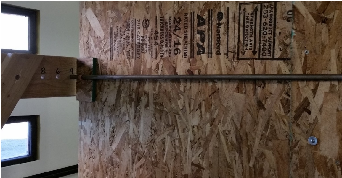
(b) Removable metal rod secures the wall through holes and eyelets
