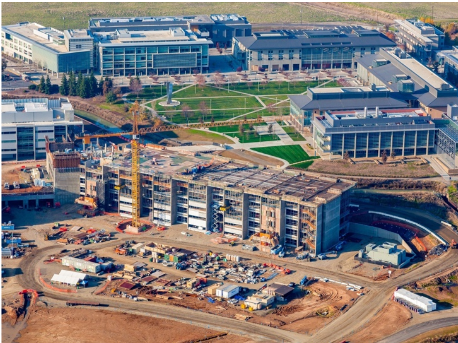
Figure 8. UC Merced Construction in January 2019 Courtesy: Merced2020 Instagram
