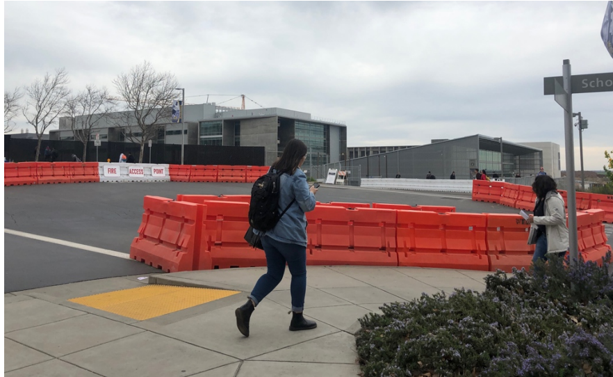
Figure 22. Construction barriers on Scholar's Lane block road access to the bridge
