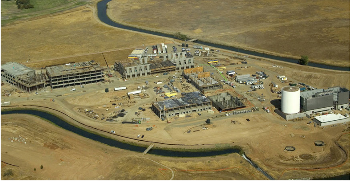
Figure 4. Aerial shot of construction on UC Merced in 2004
