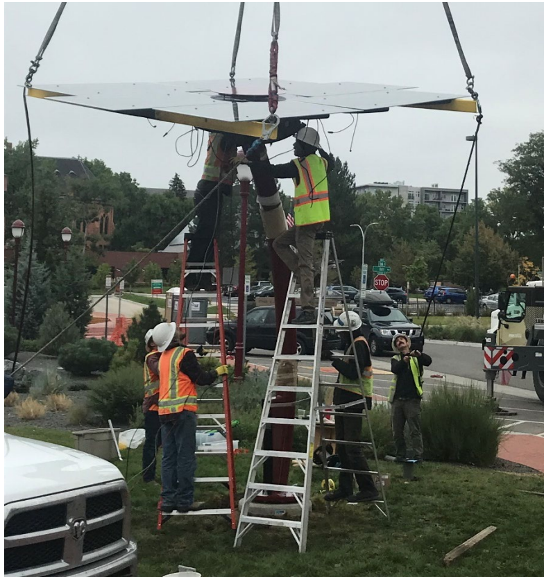
Figure 20: Installation of Solar Tree on DU Campus 4
