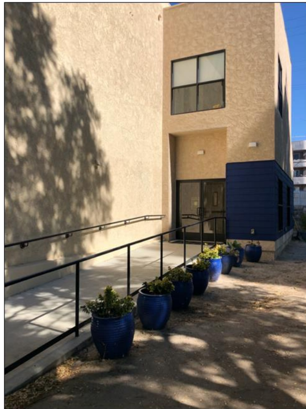
Figure 4.32: ADA-Compliant Ramp and Elevator in Middle and High School Building
