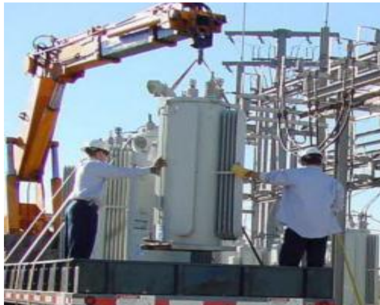
Fig. 1.2 Transformer maintenance service [10]
