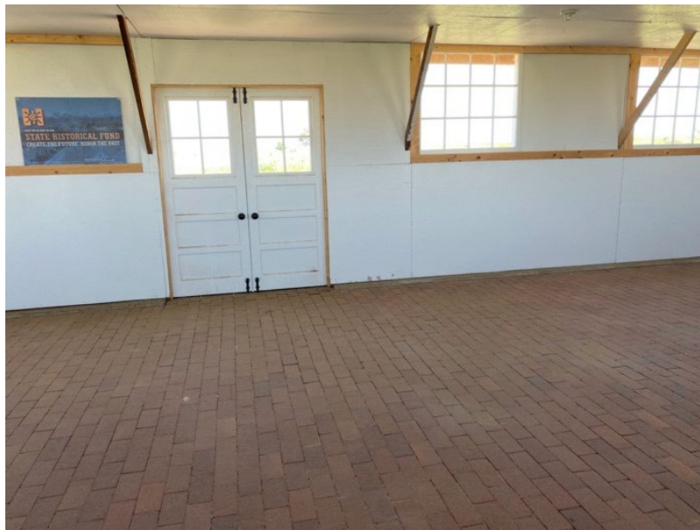
Figure 7: Interior of rehabilitated 11F recreation hall. Photo credit Megan Brown.
