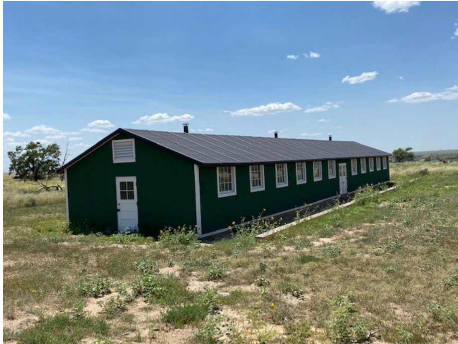
Exterior of 11F Recreation Hall. Photo credit Megan Brown.
